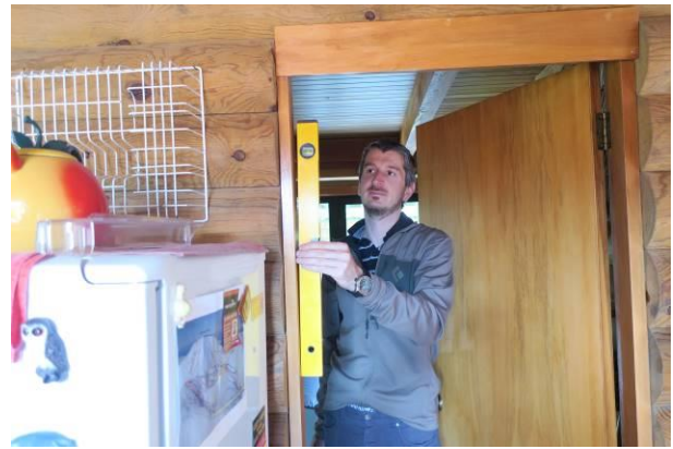
Figure 21: Sliding of logs resulting in residual drifts of the house.
