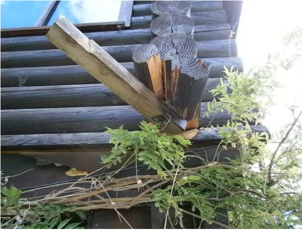
Figure 31: Crushing of bottom log.
