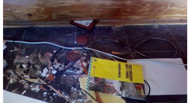
Figure 44: Trapped picture frame under sill log.
