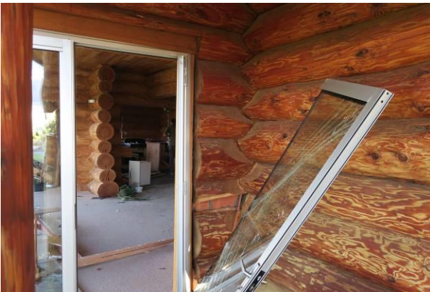
Figure 53: Typical damage to doors and windows due to large horizontal deformation.
