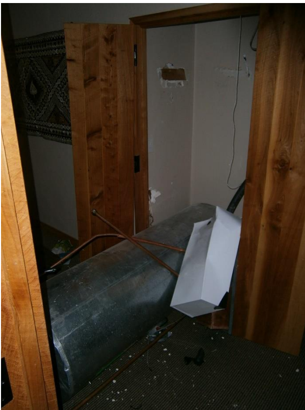
Figure 37: Damage from insufficiently restrained water cylinder.
