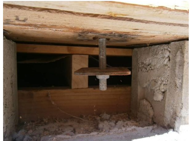
Figure 27: Fractured tie rod.
