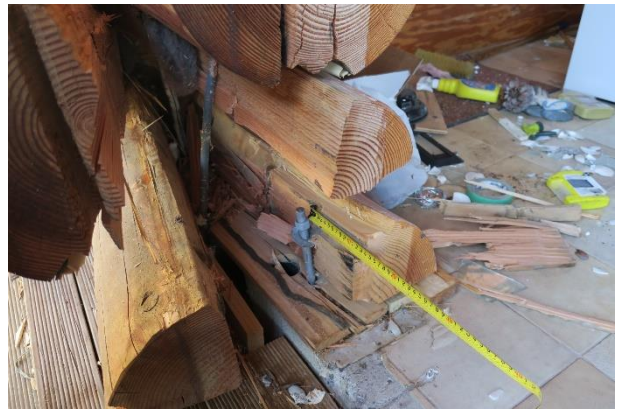
Figure 48: Splitting of logs weakened by tie rods and shear dowels.
