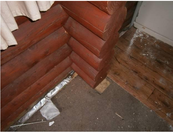
Figure 24: Sliding of the logs on suspended floor.
