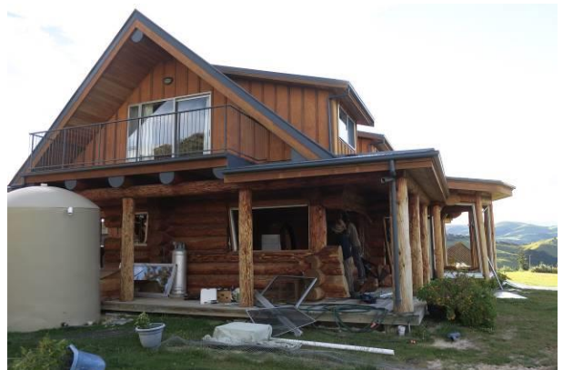
Figure 39: Two storey traditional log house with visible residual drift.
