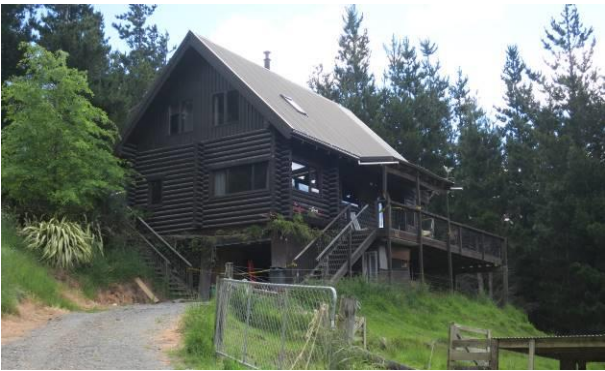
Figure 4: Two storey log house on slope with pole foundation.
