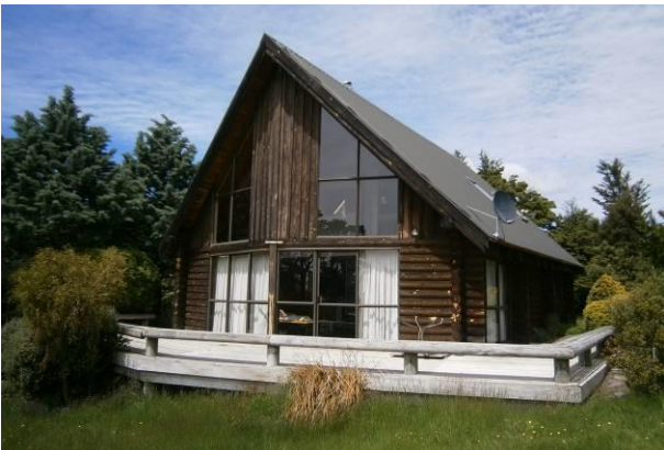
Figure 5: Two storey log house.
