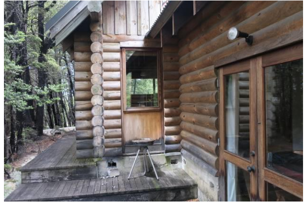
Figure 6: Two storey log house with slab on grade foundation.
