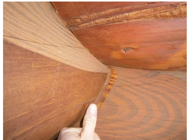
Figure 22: Sliding of the logs at corners.
