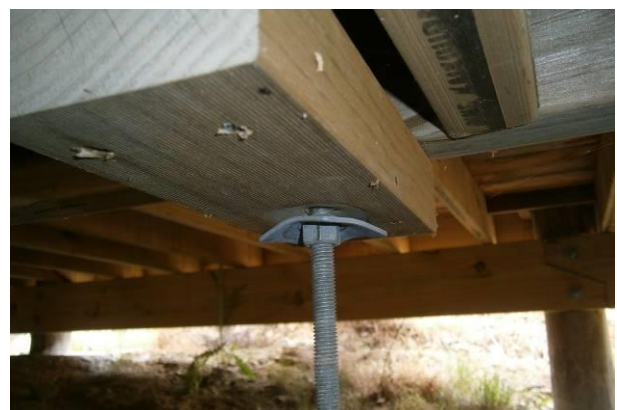
Figure 29: Bent washer and wood crushing in anchorage block.
