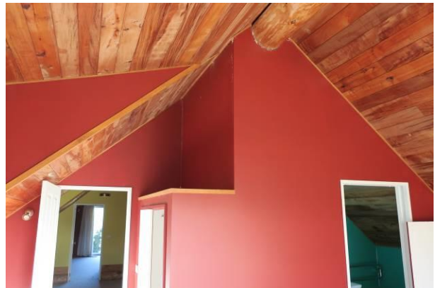
Figure 56: Damage in the upper storey was very limited.
