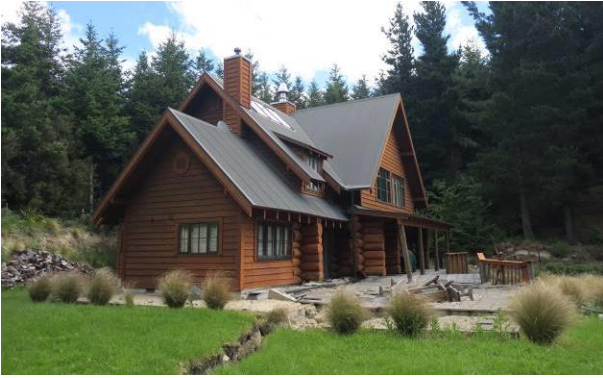
Figure 10: Two storey traditional log house with geotechnical damage.
