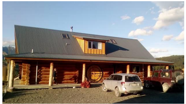
Figure 38: Two storey traditional log house.
