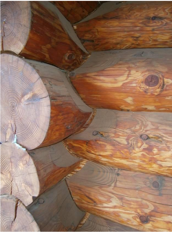
Figure 41: Permanent deformation in corner area.
