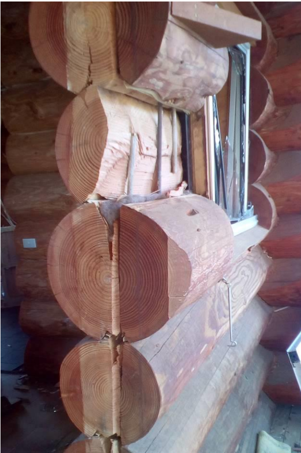
Figure 52: Splitting of log due to weakening by dowels, tie rod and vertical slot at door frame.
