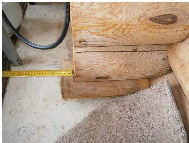
Figure 16: Sliding at the top of the bottom half-log.
