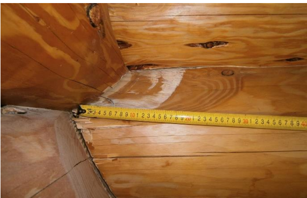
Figure 42: Permanent deformation in corner area.
