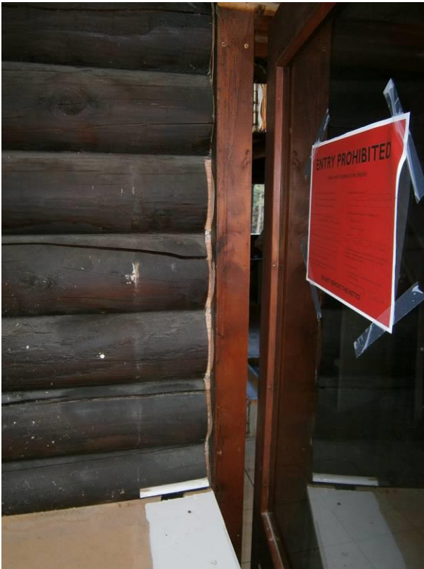
Figure 19: Localized sliding of logs.
