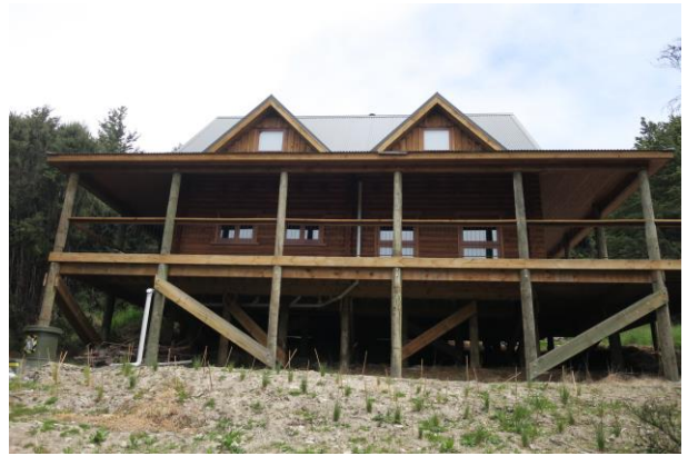
Figure 7: Two storey log house with pole foundation.
