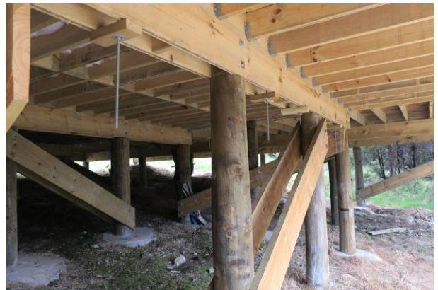
Figure 8: Pole supports with diagonal sub-floor bracing.
