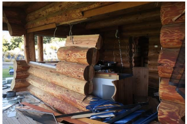
Figure 50: Wall stability failure and splitting of logs.
