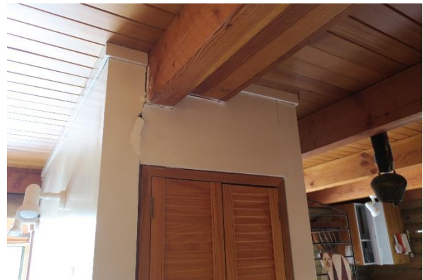
Figure 35: Typical cracking of gypsum plasterboard.
