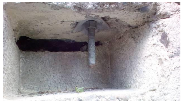
Figure 28: Bent washer in concrete pocket.
