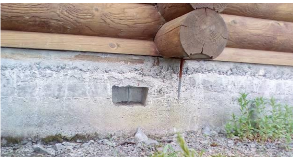
Figure 12: Typical connection details with vertical steel rods and anchorage into foundation and half log (sill log).
