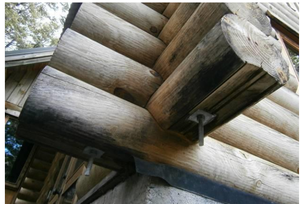
Figure 13: Typical connection with threaded rods through the logs.
