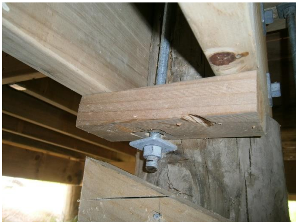
Figure 14: Typical anchorage with a timber block between floor bearers.
