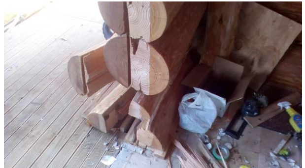
Figure 49: Splitting of bottom log weakened by vertical slot at door frame.
