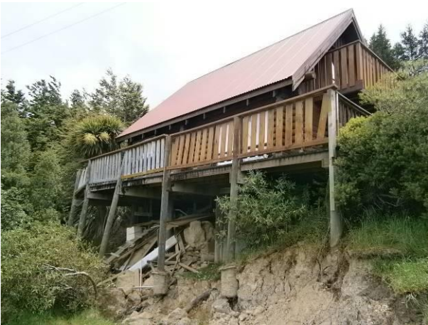
Figure 11: Two storey log house on slope with pole foundation with slope stability failure.
