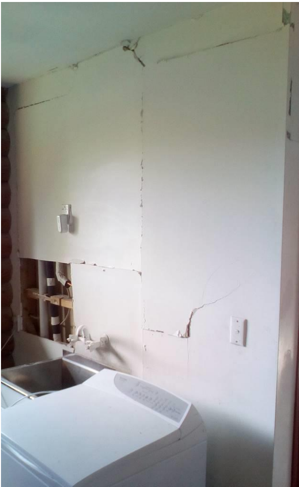
Figure 36: Typical cracking of gypsum plasterboard.
