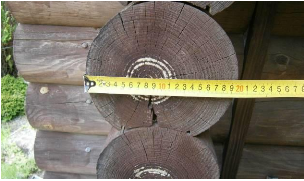
Figure 2: Typical machined logs.
