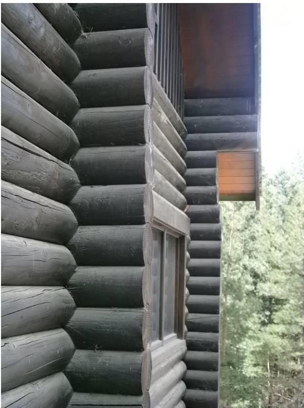
Figure 20: Sliding of logs resulting in residual drifts of the house.
