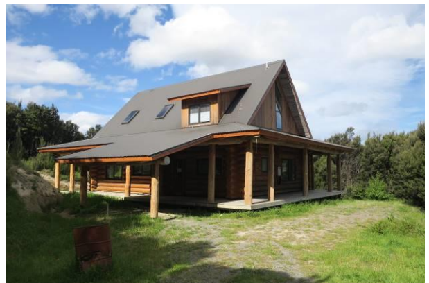
Figure 9: Two storey traditional log house.
