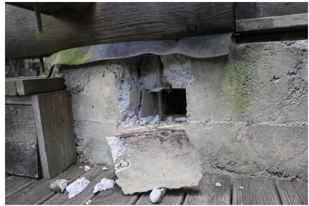
Figure 26: Damage to pocket in concrete foundation due to missing reinforcement.
