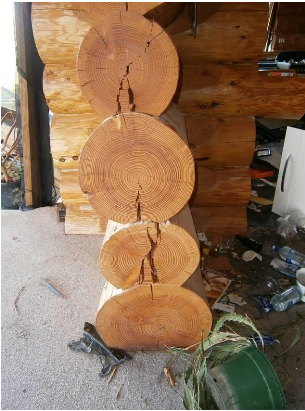
Figure 46: Initiation of splitting in logs, undamaged bottom log.
