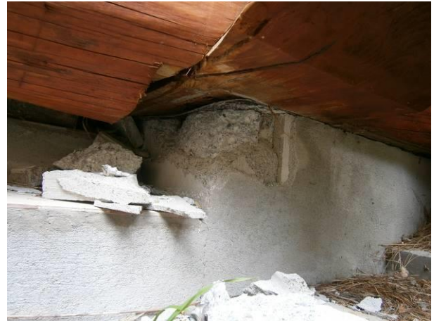
Figure 34: Cracking and spalling of concrete due to large compression forces.
