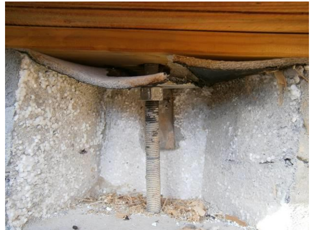
Figure 45: Yielding failure or fracture of tension rod.
