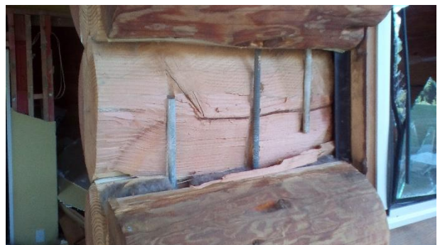
Figure 51: Splitting of log.
