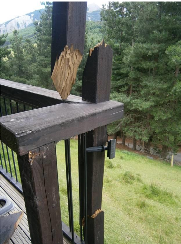
Figure 25: Fracture of veranda post due to excessive lateral movement.
