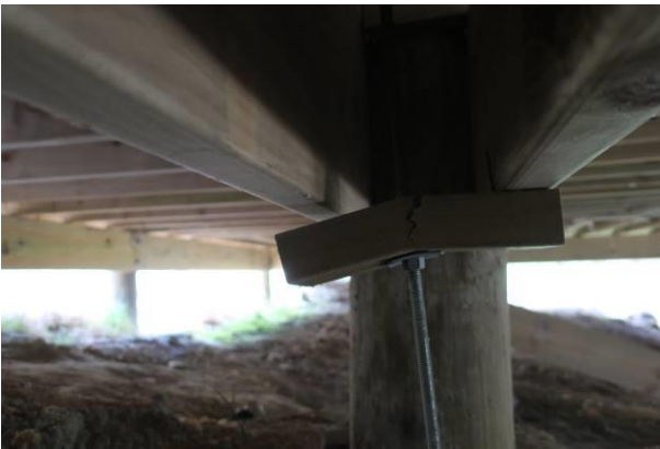
Figure 32: Failure of timber anchorage block.
