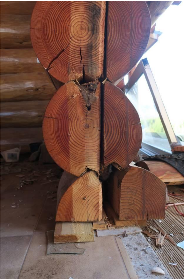
Figure 47: Splitting of bottom log.
