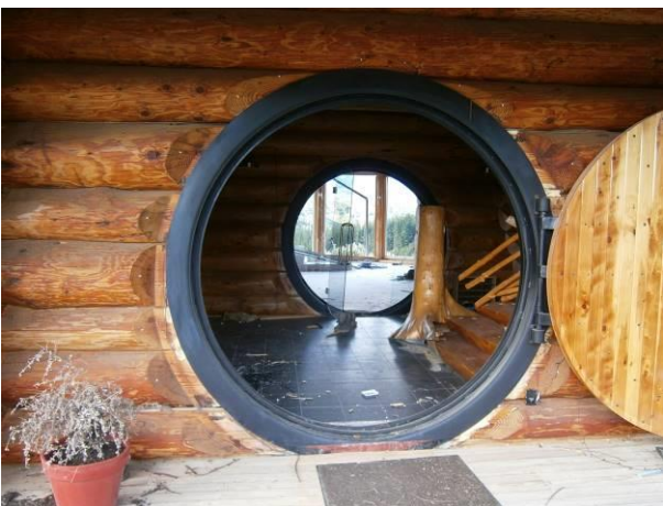
Figure 43: Large deformation around very stiff circular door frame.
