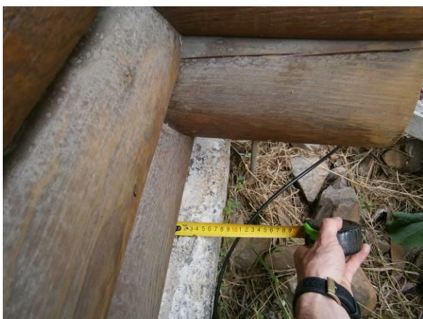
Figure 15: Horizontal sliding of the house.
