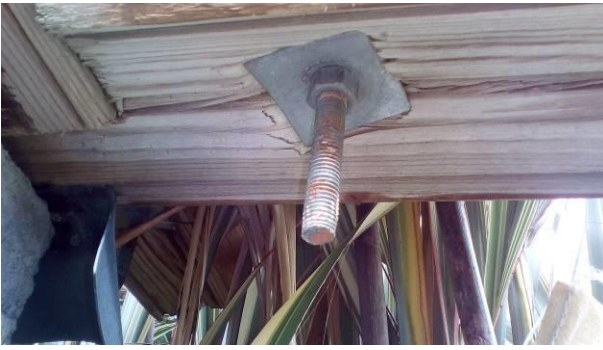
Figure 30: Bent washer and wood crushing in bottom log.
