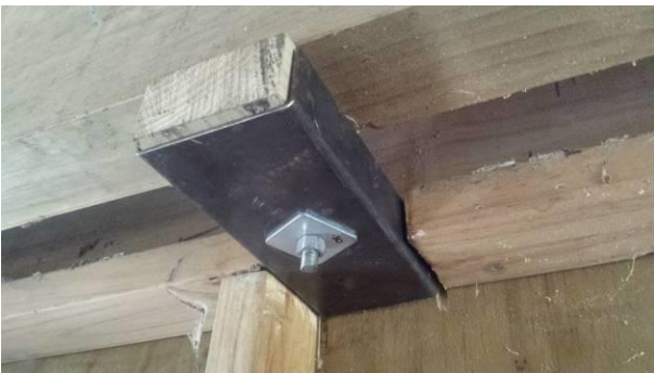
Figure 33: Reinforcement of timber anchorage with a steel profile.
